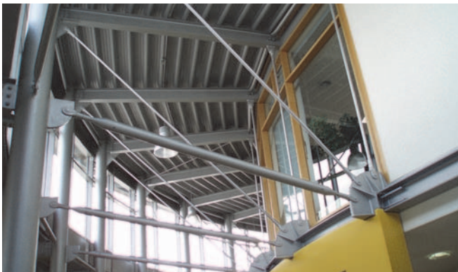
Bracing between an exterior steel column and an interior steel beam
