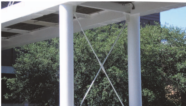
Cross-bracing with a cross coupler
